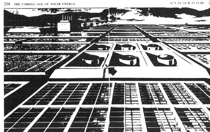
Artist's impression of a solar power plant. Arrow points to a human figure, dwarfed by its surroundings. A 1,000 MW fossil-fired or nuclear plant can be built on a few acres; a 1,000 MW solar plant would need 50 square miles of collecting area. No technological advance can ever change the dilute solar influx of 1 kW/m<sup>2</sup>.
