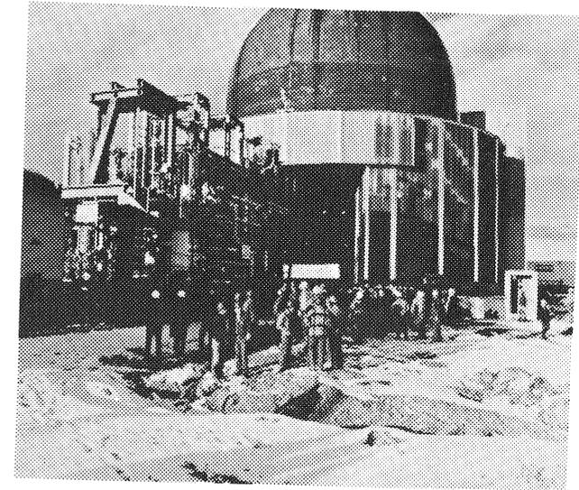
The LOFT (Loss of Fluid Test) facility in Idaho is designed to provide accurate tests of the effectiveness of emergency core cooling during a large simulated loss-of-coolant accident. The first of a series of tests, in March 1976, was a complete success.
